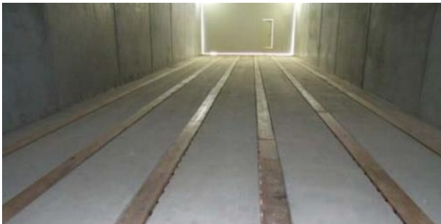
Above: Custom In-Vessel Forced Aeration Compost Tunnel
